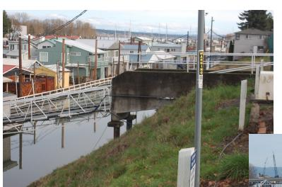
overbuild. These services branch perpendicular to the levee and emerge from underground beneath each access ramp. These services will need to be preserved or upgraded as part of any substructure project.
